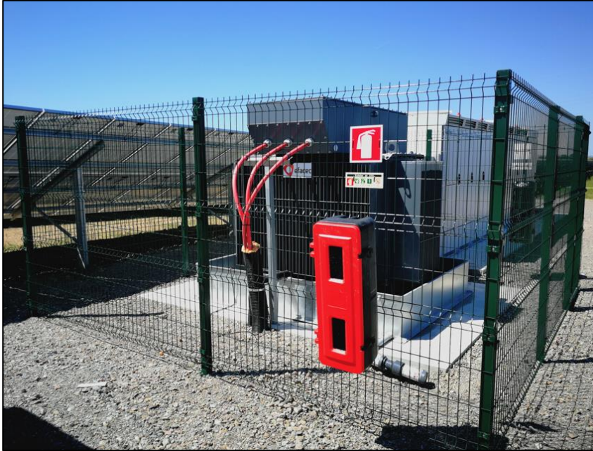
Plate 4-11. Typical transformer compound fencing
