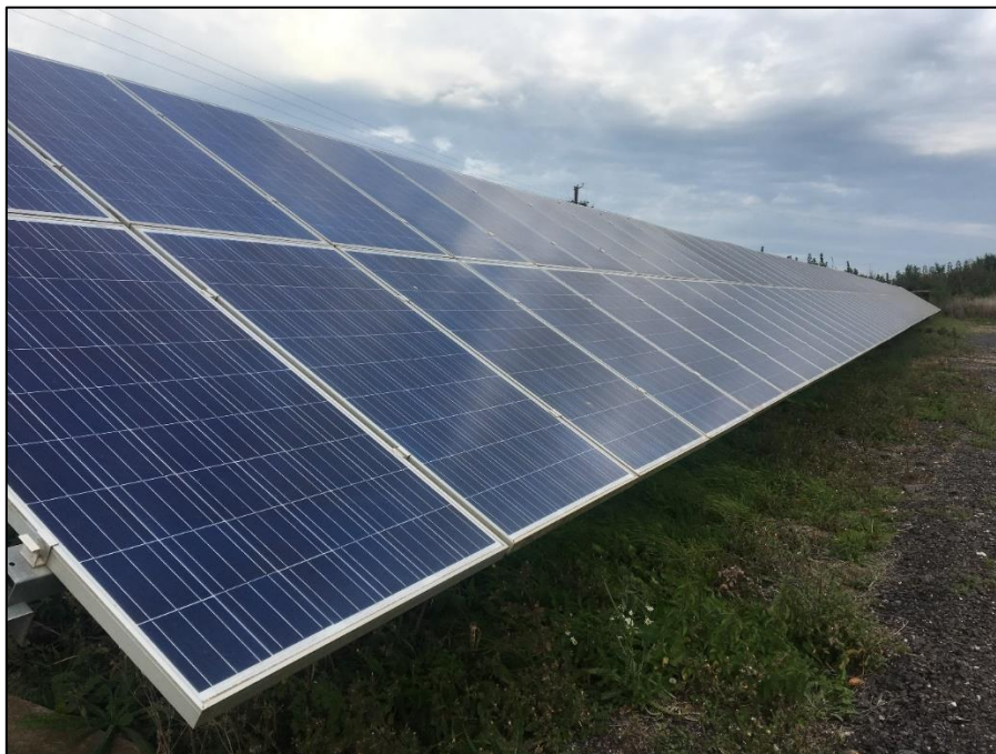
Plate 4-3. Solar panels with south facing configuration
