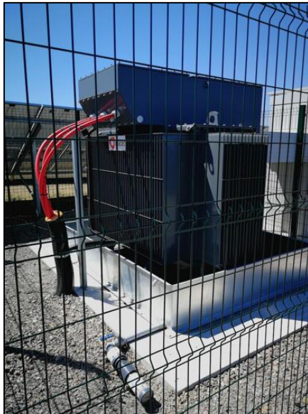
Plate 4-6. Typical outdoor transformer
